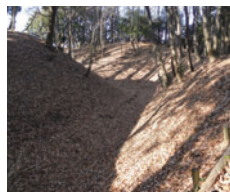
Moat and Embankment
